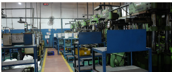
CURING LINE, HYDRAULIC PRESSES
